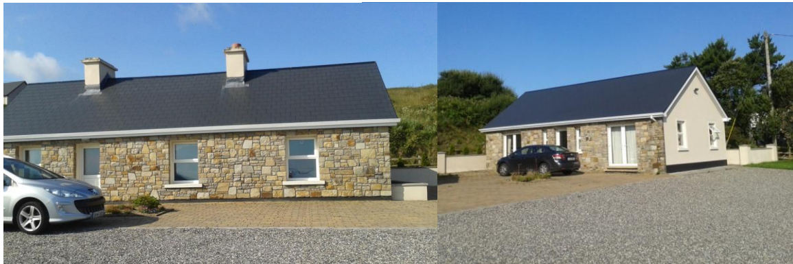
The old house with chalet bedrooms on the right
